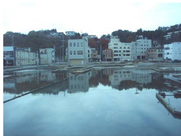
Fig. 9: Land subsidence and water logging (Kesennuma)
