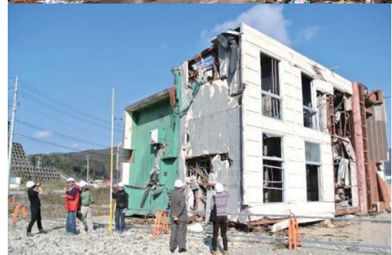
Tsunami damage by the 2011 Tohoku-Oki Earthquake
