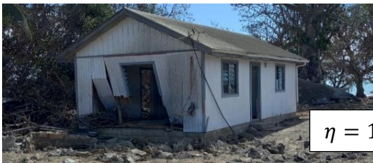
Fig. 1. Damages to the CRH at different inundation depths
