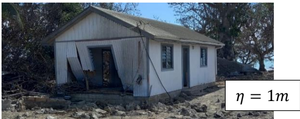
Fig. 1. Damages to the CRH at different inundation depths
